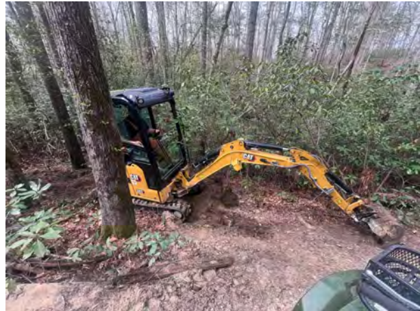
Excavating at Lake Lurleen State Park
